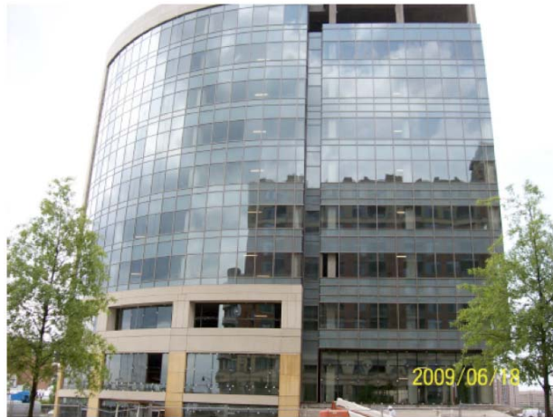
Figure 1: Curtain Wall System
