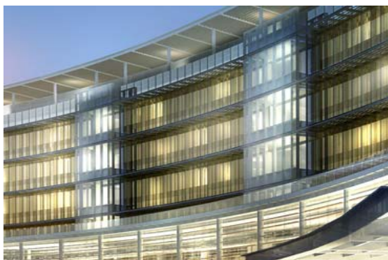
Figure 1.2- Windows on Curtain Wall
