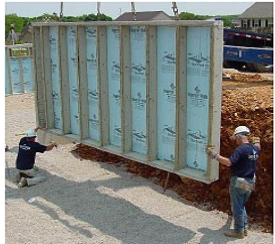
Figure 3.6 - Pre Cast Foundation Wall Being
