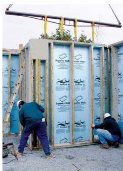
Figure 8.2 - Placement of Pre-cast Foundation Wall
