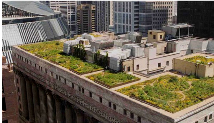
Figure 4.1 – Green Roof on Top of Chicago City Hall
