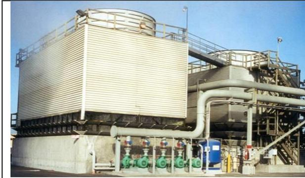
**Figure 7-1.1 - Cooling Tower** (Courtesy of Zetacorp)
