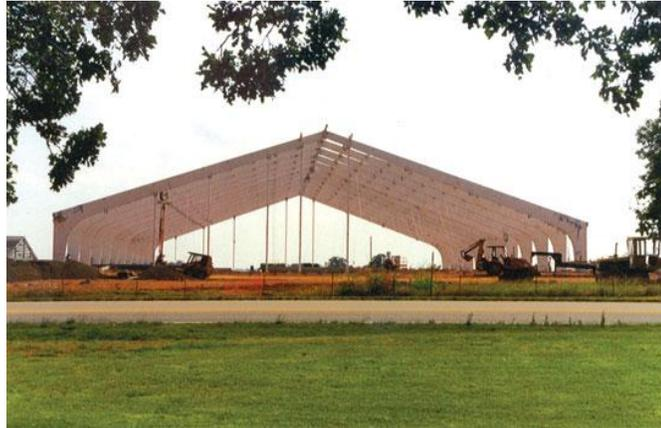
**Figure 9-1.1 - Glulam Arches** (Courtesy of Structural Mag)
