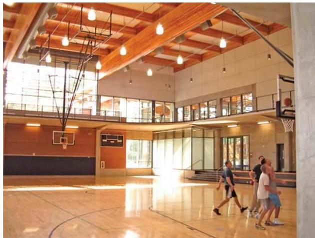
Figure 5-2: Gymnasium with glulam structural system. Courtesy of Structure Mag
