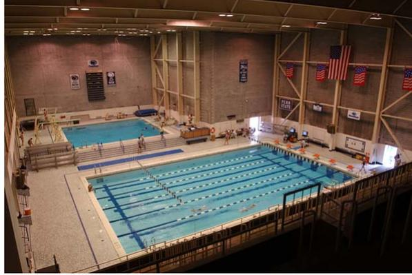
Figure 5-1: Natatorium with steel structural system. Courtesy of Penn State
