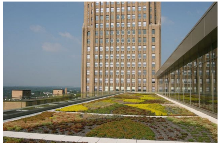
Figure 60: Extensive Green Roof Installed in Allentown, PA
