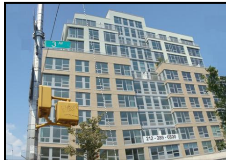
Figure 4: Neighboring Luxury Condominiums
