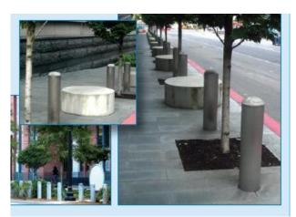
Figure 10.14 – Bollard and Tree Site Barrier. Credit to FEMA 430
