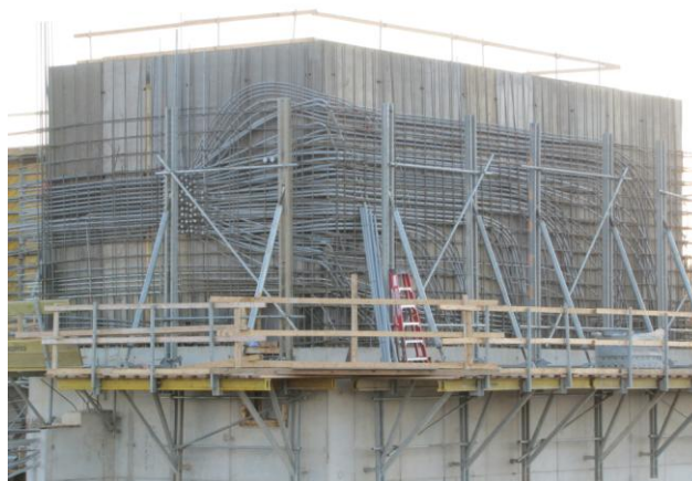
Figure 3: View of the Conduit in the Theatre Walls
