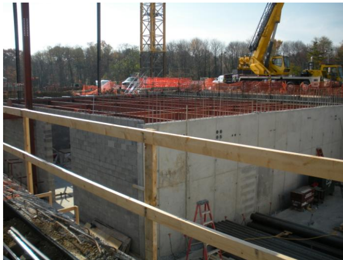
Figure 1: View of all 3 Structural Elements in Basement
