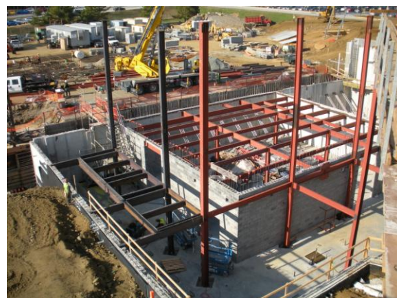
Figure 2: View of Structural Steel in Humanities Section
