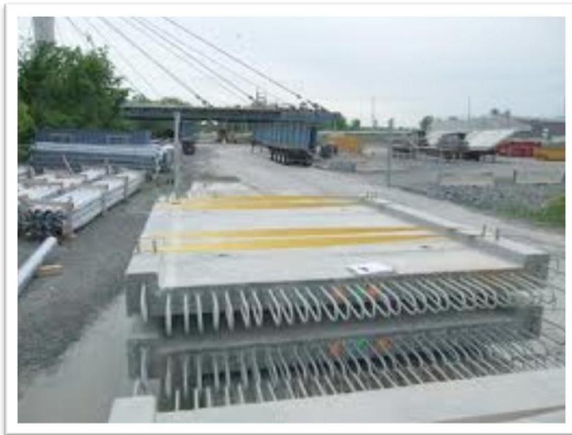
Figure 4 - Prefabricated Floor Panels
