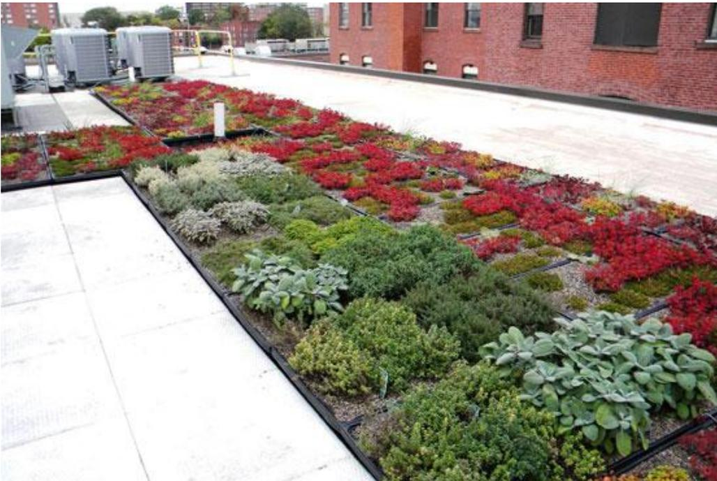
**Figure 48** Typical installation of a 4" deep extensive GreenGrid system.
