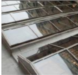
Dining Area Roof
