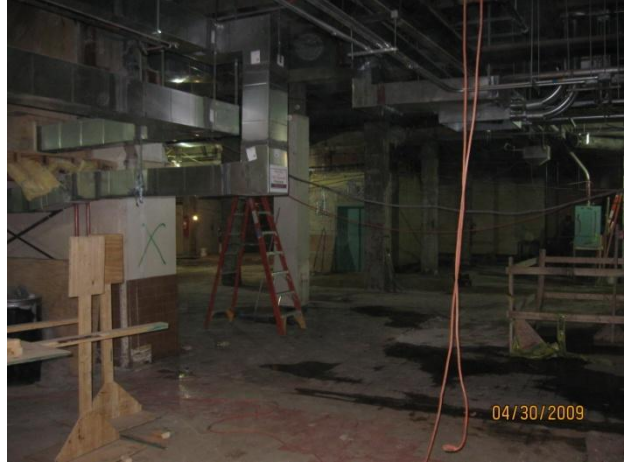
Kitchen Area Demolition
