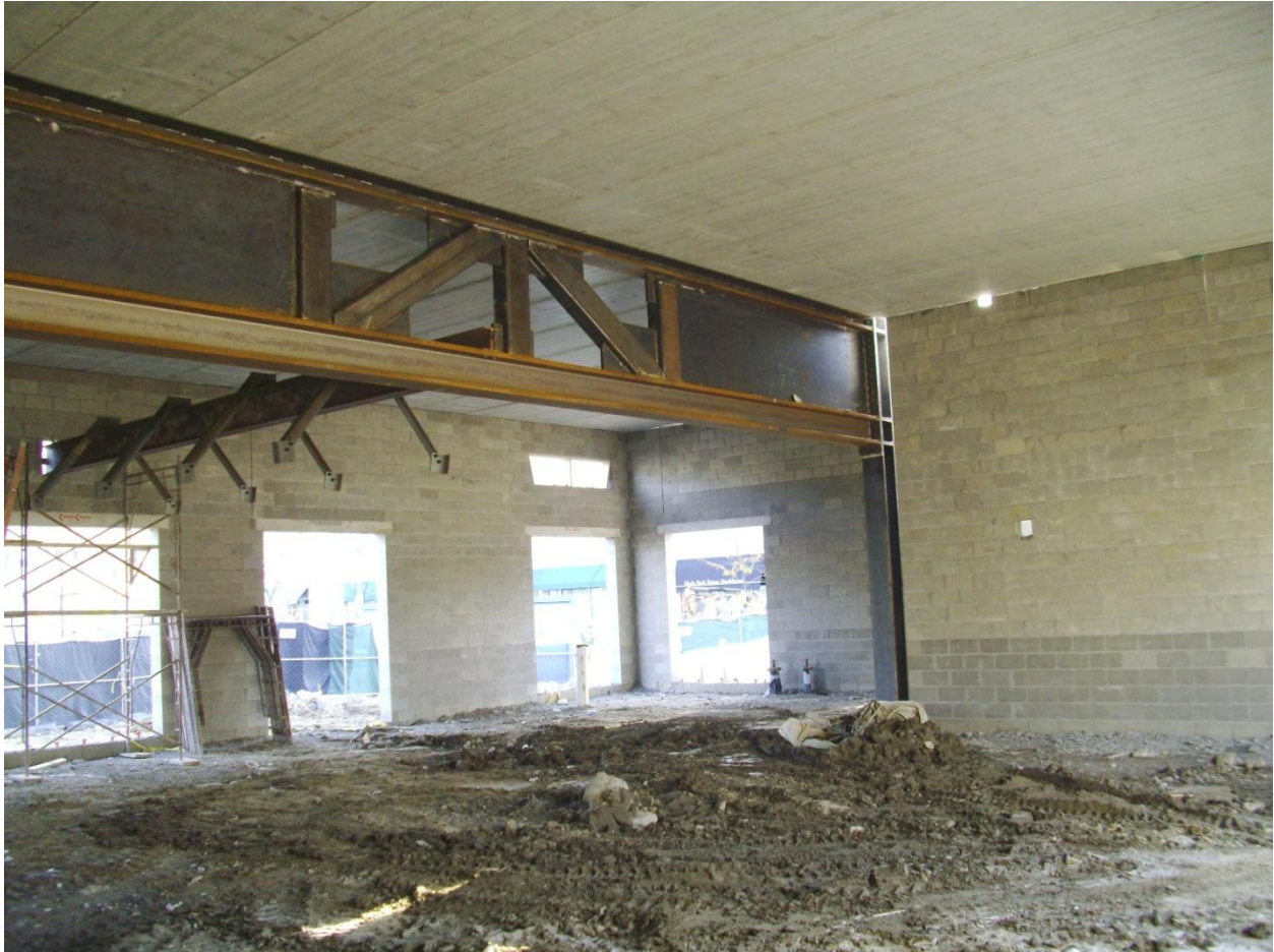
Steel Truss Over Meeting Room
