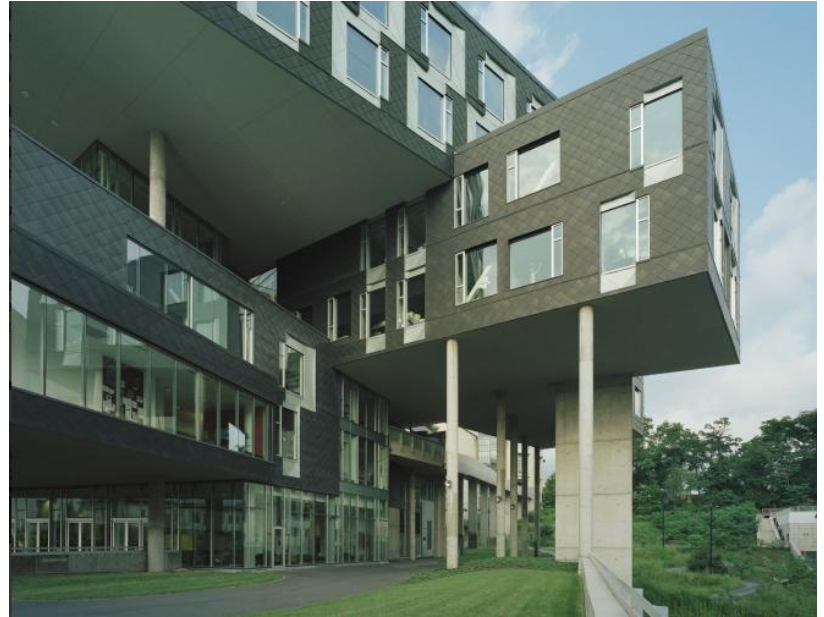
Figure 8 – South cantilever of the 6 th and 7 th floors.
