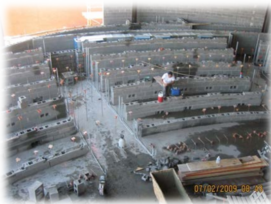
Figure 4: Installation of lecture hall structure
