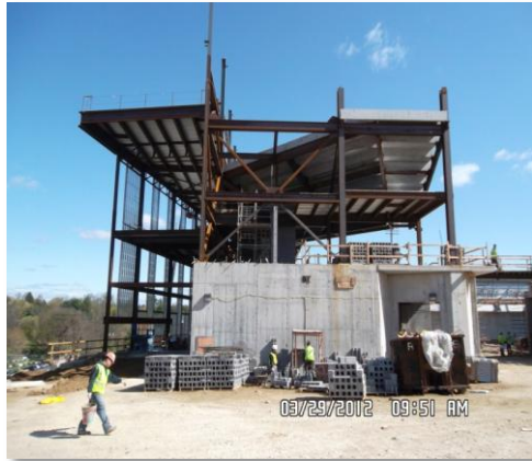
Figure 3 Section of TA Structure, taken by Ryan Simmons
