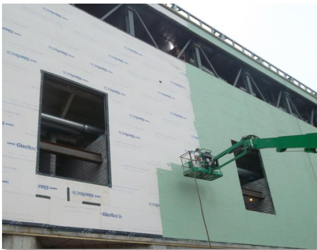
Figure 6 West Air Vapor Barrier, taken by Derek Stoecklein
