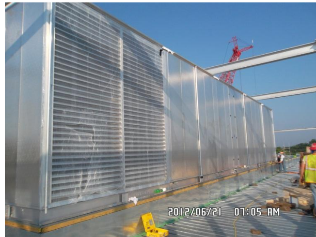
Figure 4 Custom AHU for TA, taken by Derek Stoecklein
