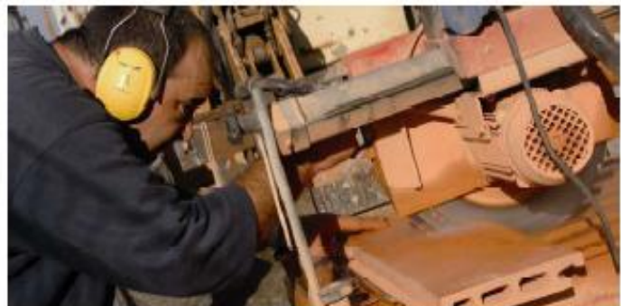
Field Cutting Terra Cotta Panels
