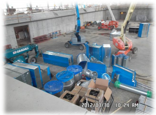
Figure 14 photo of duct work on the bowl floor, taken by Derek Stoecklein
