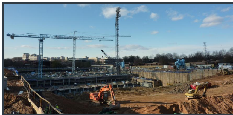
Figure 1: Construction of the Reston Station Garage
