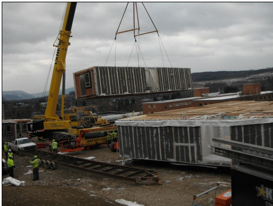
Figure 39 Modular Unit Moved by Crane
