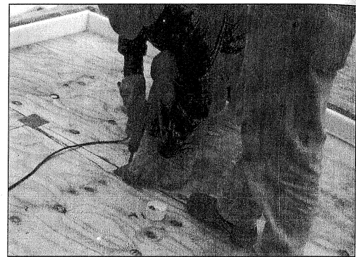
7.13 Connecting plywood panels together. Photo by Madan Mehta.
