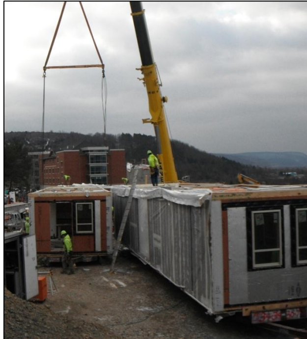
Figure 38 Modular Unit Crane Rigging
