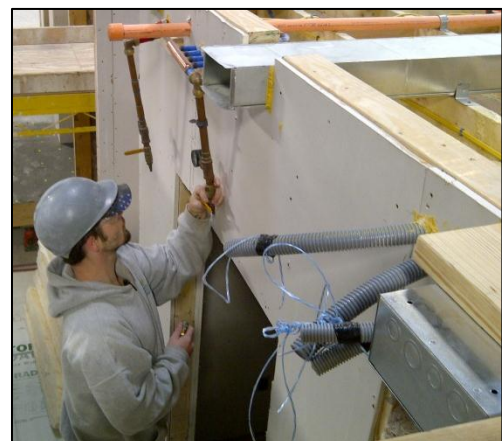
Figure 7 CMU Modular Unit MEP Rough
