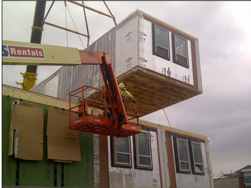
Figure 40 Men on Lifts Adjusting the Modular Unit
