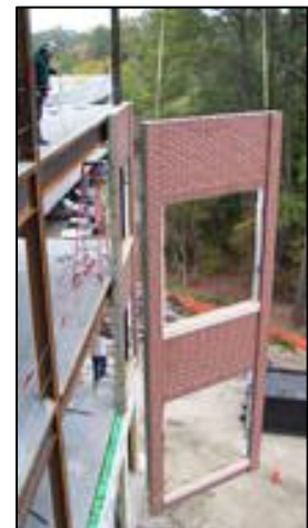
Figure 22 Panelized Thin Brick Facade Courtesy of Advanced Exterior Systems
