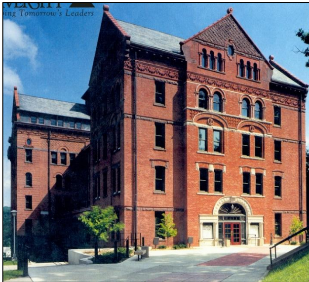
Figure 23 North Hall Library Courtesy of Mansfield.edu
