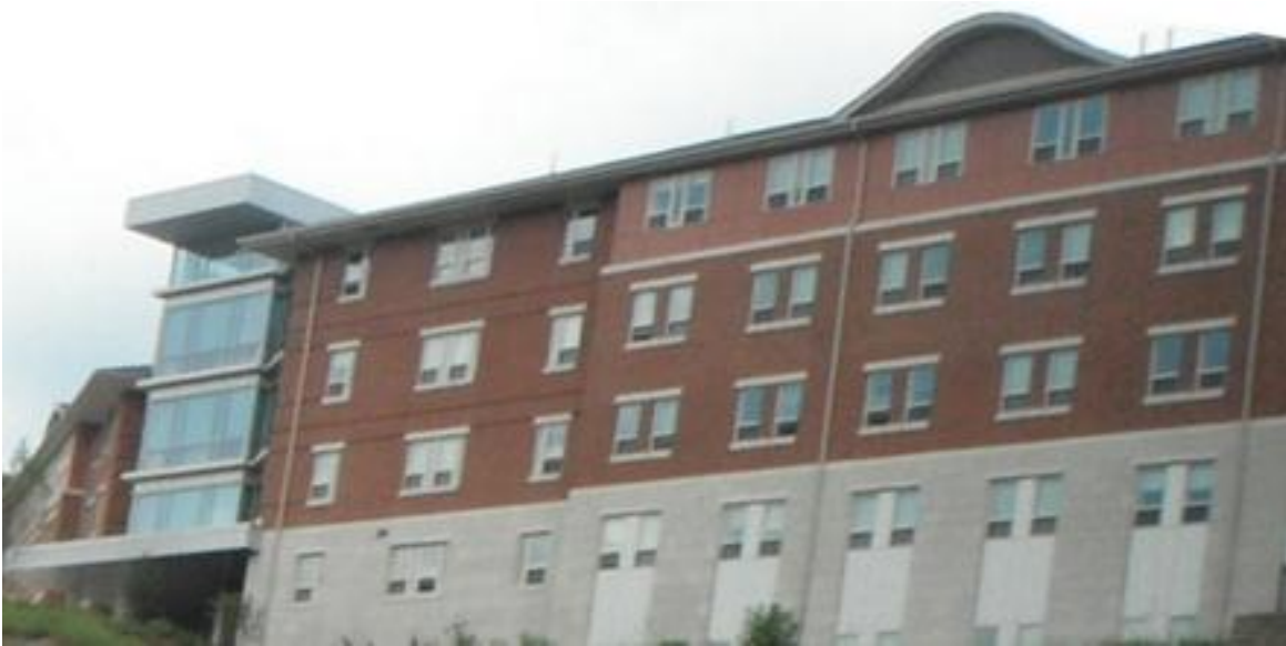
Figure 21 Masonry Façade Phase 1 Dormitory
