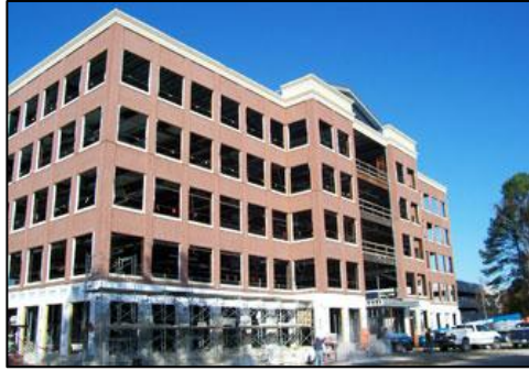
Figure 30 Convergence Center Courtesy of Advanced Exterior Systems
