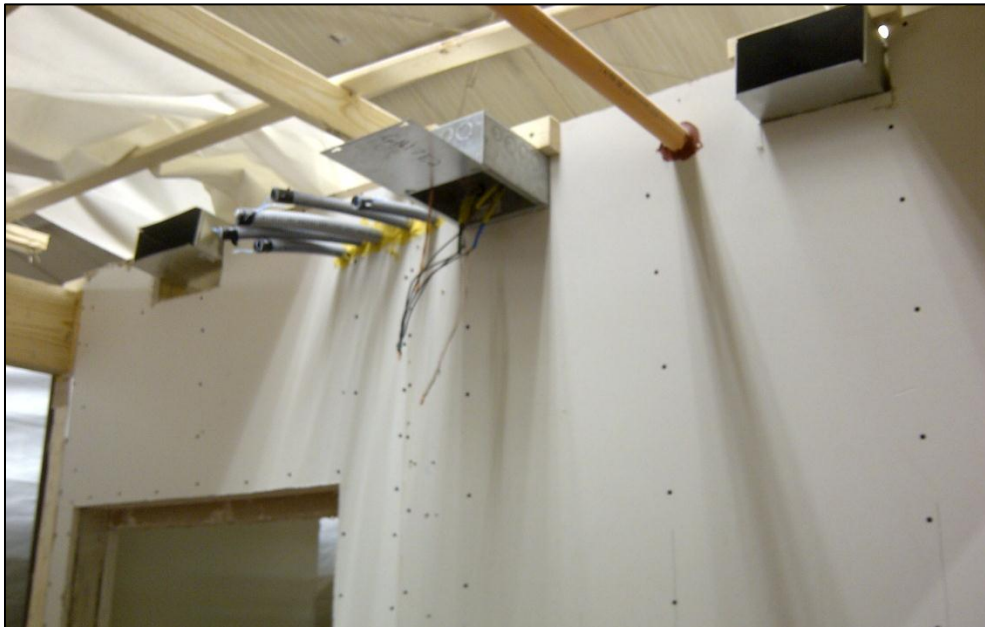
Figure 20 MEP Hallway Connections
