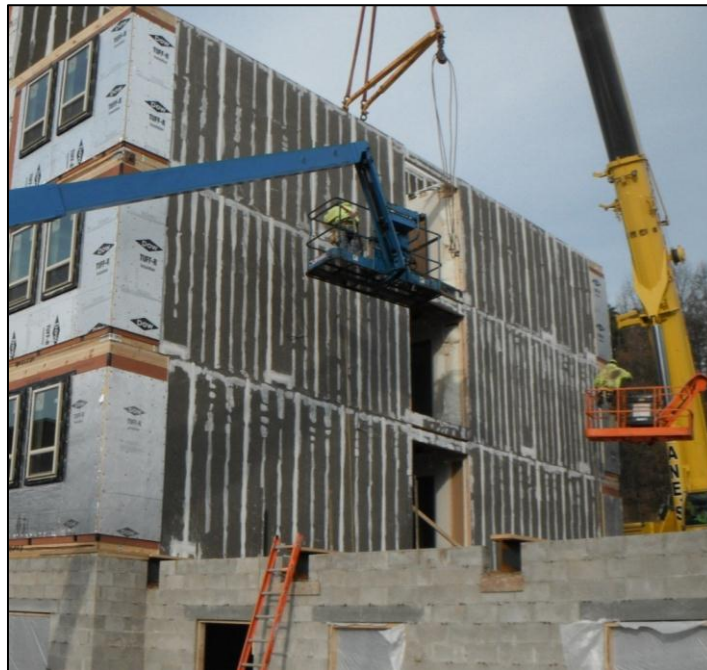
Figure 41 Anchoring Modular Unit
