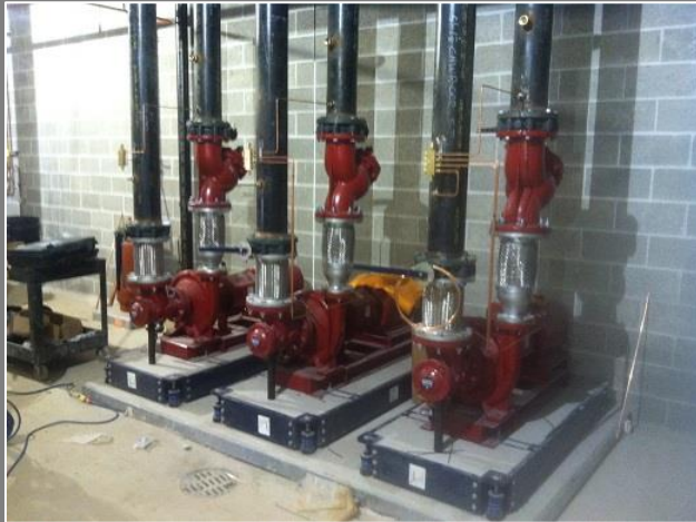
Chilled Water Pumps (3-25HP)
