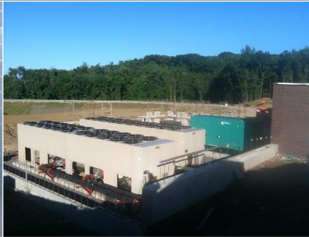
Mech. Yard – 2 Chillers, Diesel Generator & Utility Transformer
