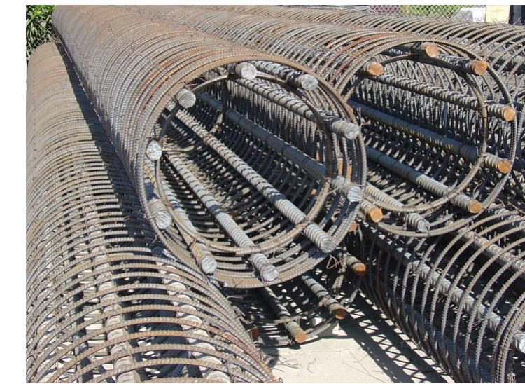
Picture Provided by www.rebarsupply.net
