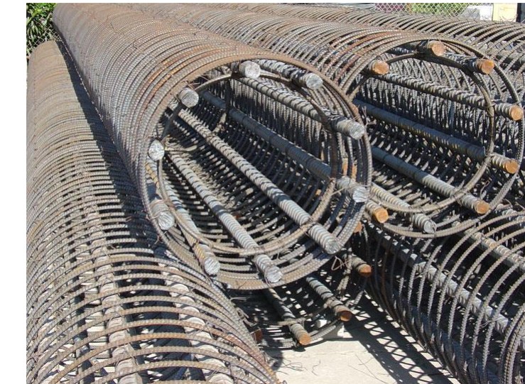
Picture Provided by www.rebarsupply.net
