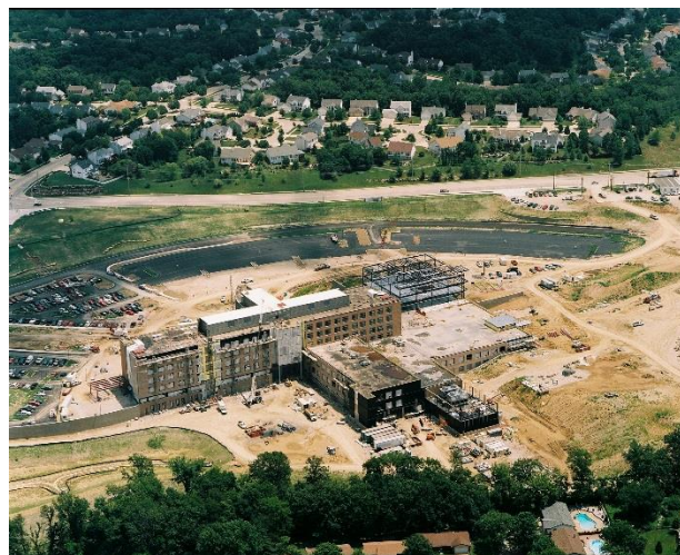
Figure 2: Aerial view showing proximity to residential areas
