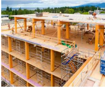
(a) CLT Building. Source: woodwindowstoday.blogspot.com
