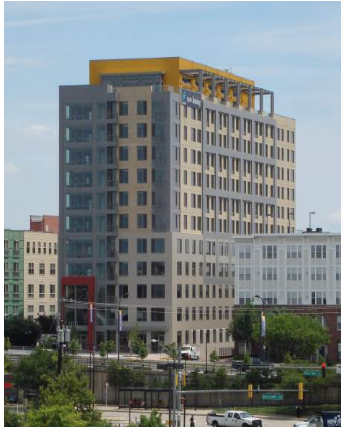
Figure 1.2: View of 11141 Georgia Ave
