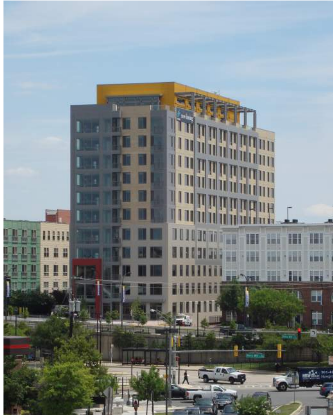
Figure 1.2: View of 11141 Georgia Ave
