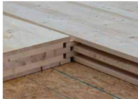
(b) Double Spline Connection. Source: CLT Handbook
