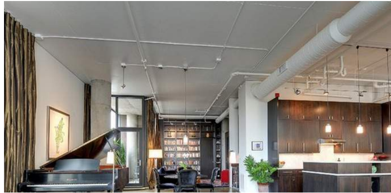
Figure 5.1: Example of exposed mechanical equipment. Source: Houzz.com
