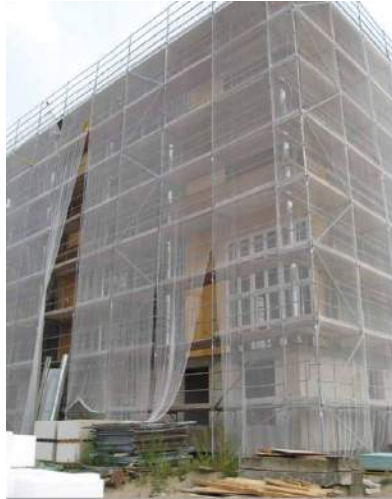
Figure 2.11: Moisture Protection of CLT During Construction. Source: CLT Handbook
