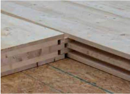
(b) Double Spline Connection. Source: CLT Handbook
