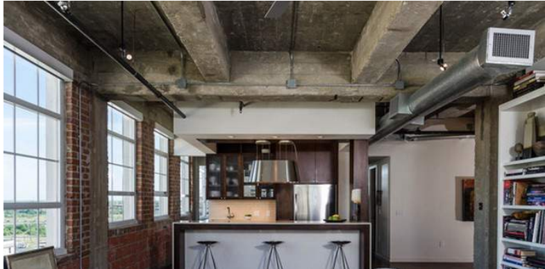
Figure 5.2: Example of exposed mechanical equipment. Source: Houzz.com
