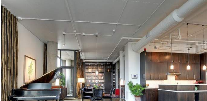
Figure 5.1: Example of exposed mechanical equipment. Source: Houzz.com
