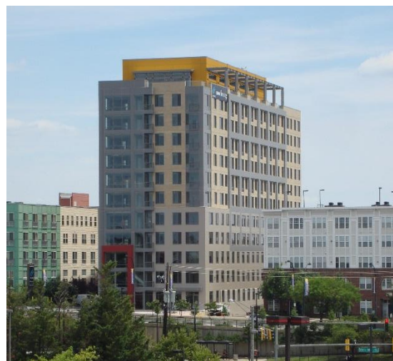
Figure 2: View of Building from nearby mall garage
