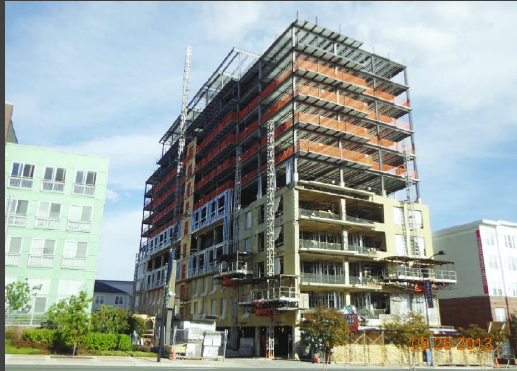
Image Source: Whiting Turner Progress Photos
