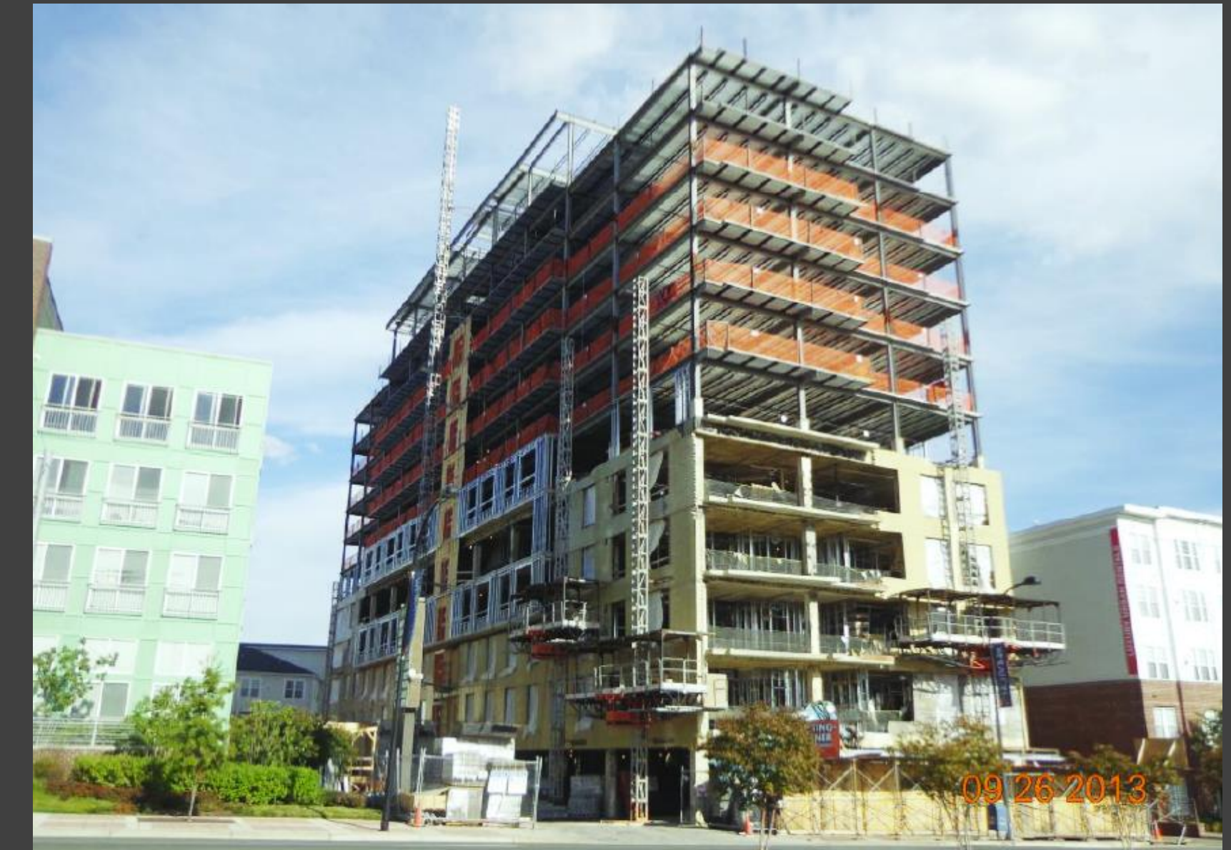
Image Source:Whiting Turner Progress Photos
