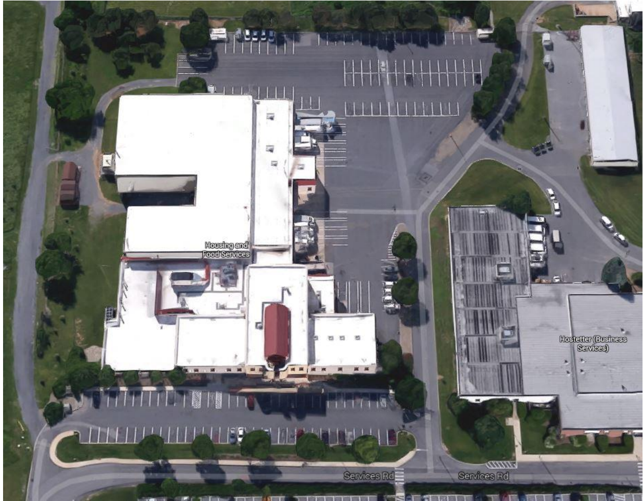
Figure 3 – Aerial View of HFS Warehouse and Bakery
