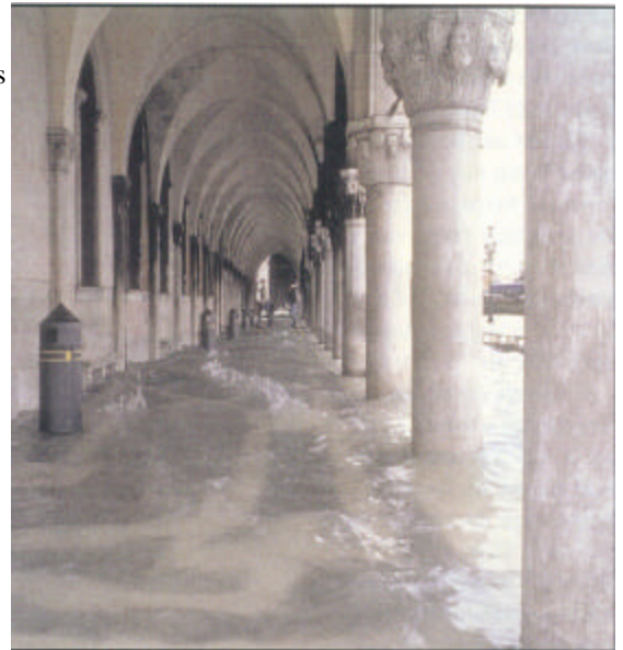
THE PORTICO of the Doge's Palace has suffered long-term damage from repeated flooding.
