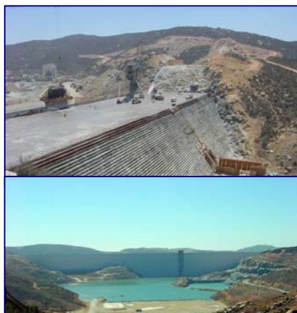
Figure 10 Olivenhain Dam, Upstream Face
