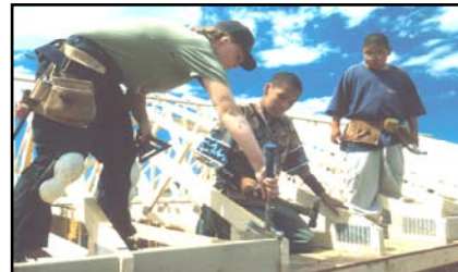
Work side by side with an Indian community in a “barn-raising” style construction process
